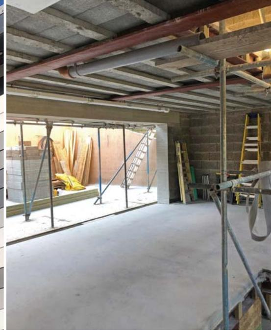
Figure 5: Beam-and-block floors bearing directly onto the Durisol walls.
